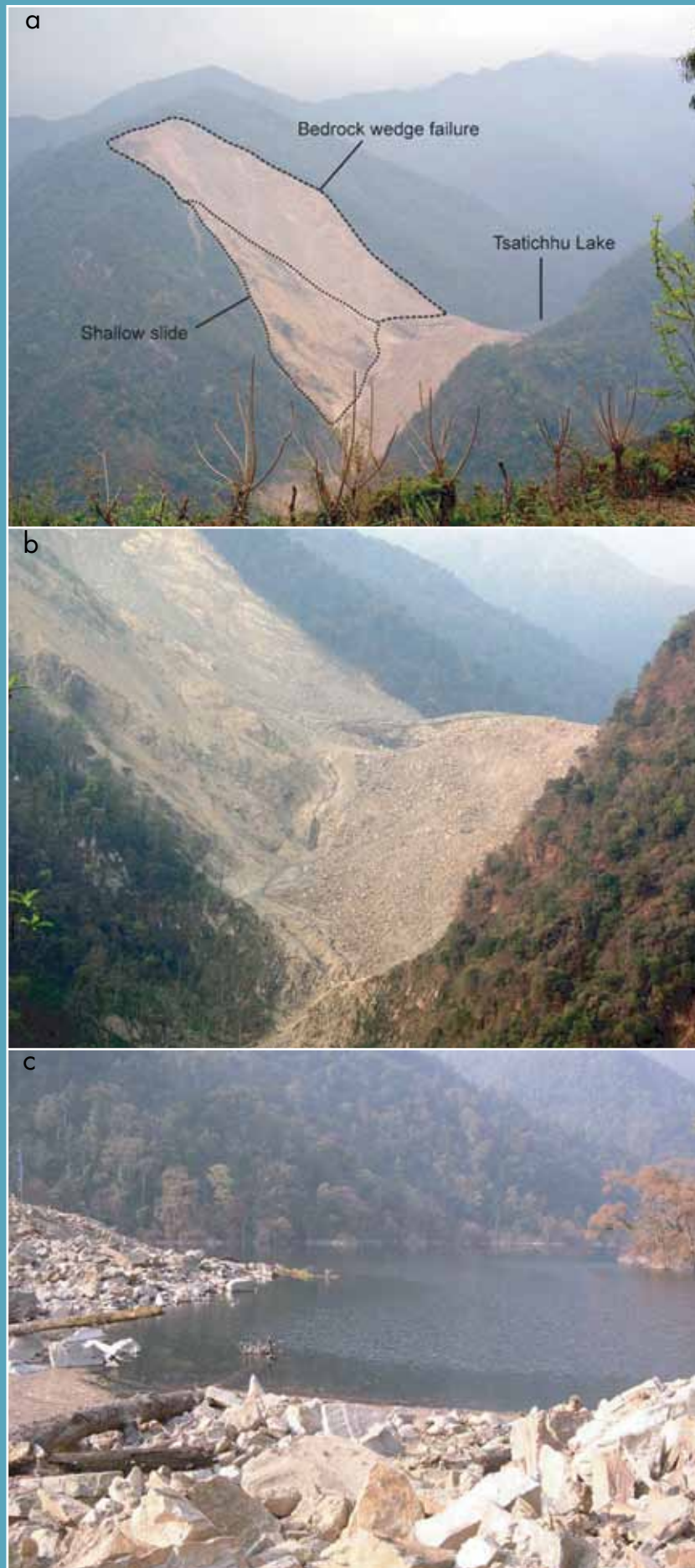
Figure 21: Tsatichhu landslide dam: a) the area at the source of the landslide; b) detailed view of the dam; c) Tsatichhu Lake
