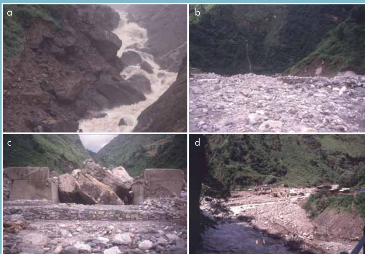
Figure 20: a) Bhairabkunda Khola a few days after the LDOF; b) debris deposited by the LDOF; c) large boulders trapped at the highway bridge; d) Larcha village destroyed by the flash flood
